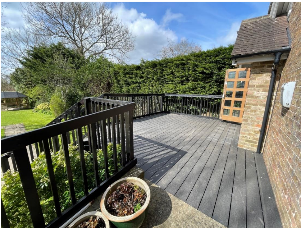
FIGURE 8 NEW COMPOSITE DECKING AT THE QUEEN'S HALL, SAM HEYNES 2022
