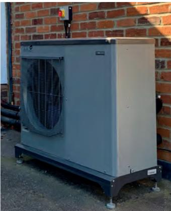
The external unit is a NIBE F2040-12, a Scandinavian design so it has no problems heating with cold external temperatures.
