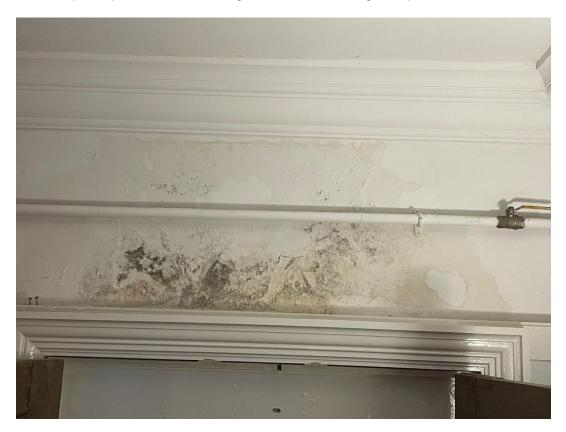
The other area of damp is in the second lobby under the war names. You can see from the picture below the wooden panelling is starting to bulge slightly and so needs to be removed and the wall be damp proofed.
