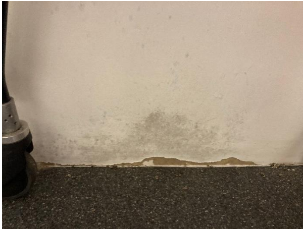
Signs of damp at floor level along external walls.
