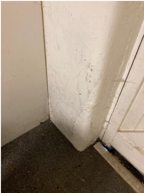
Damp to the internal door frame (left and right sides)
