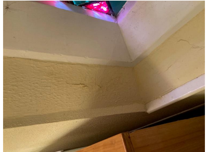
Signs of repair required around both windows, possibly caused by damp plaster.
