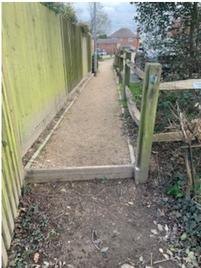
Condition of footpath March 2021, S Ockenden, 2021
